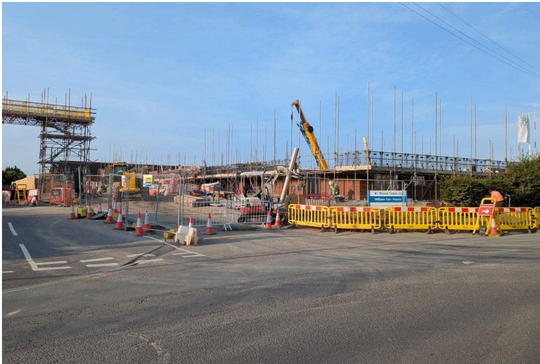
The brownfield site at William Farr House is being redeveloped to provide extra-care affordable housing. Photo: Shropshire Council
